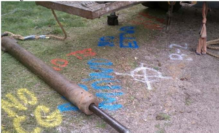
Dig Alert markings on ground near boring B-2
