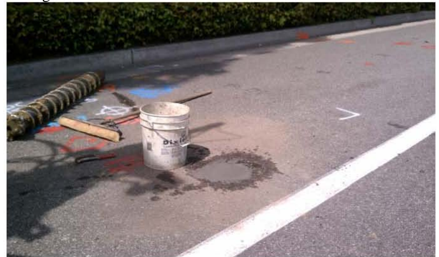
Asphalt patch after borehole completion
